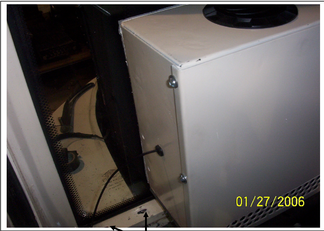
Holes marked for drilling.
